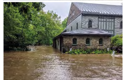
Flooding during Tropical Storm Isaias in 2020, photo credit Jamie Stewart
