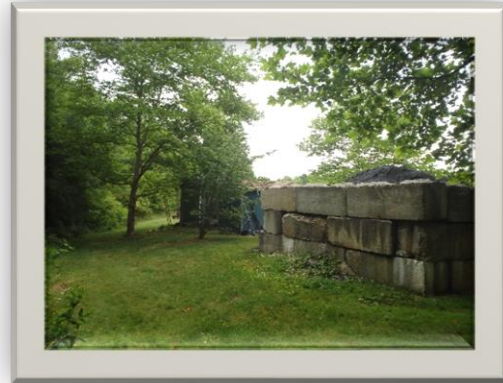
Corner of Public Works Storage
