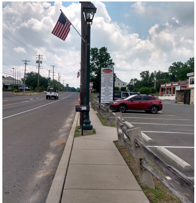
A narrow sidewalk and lack of buffer between the road and sidewalk create an unfriendly pedestrian environment.
